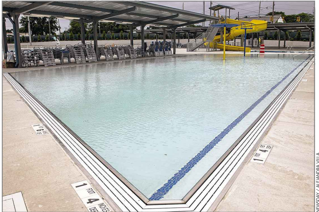
The fire marshal's office on June 29 found violations at the renovated pool at Clinton G. Martin Park.
